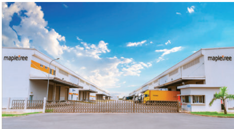
Mapletree Logistics Park Bac Ninh Phase 3
