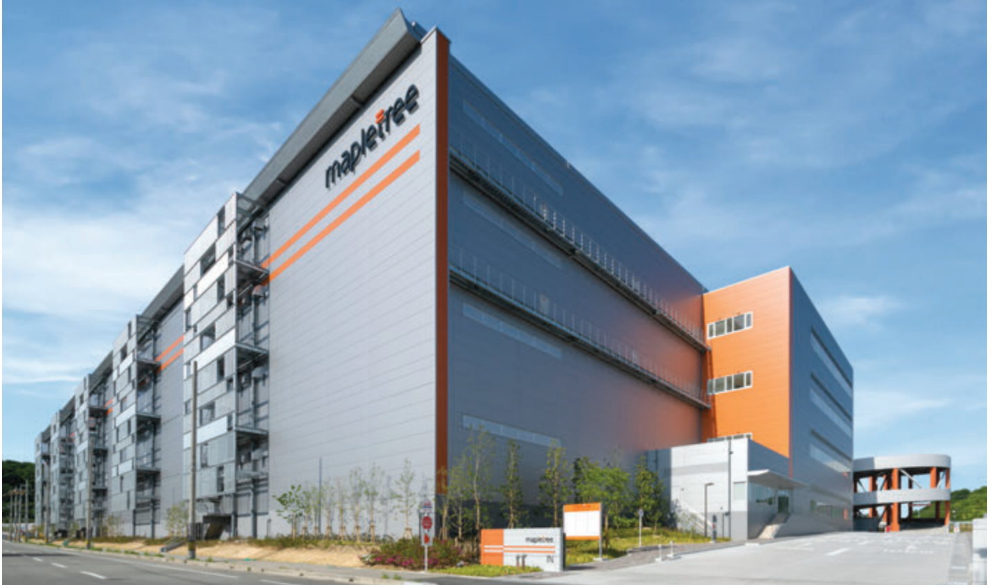
Mapletree Kobe Logistics Centre
