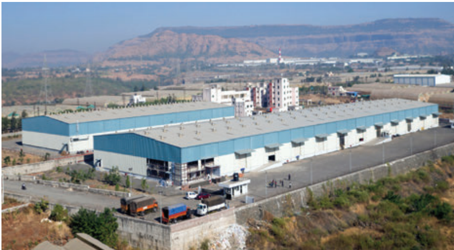
Mapletree Logistics Park Talegaon
