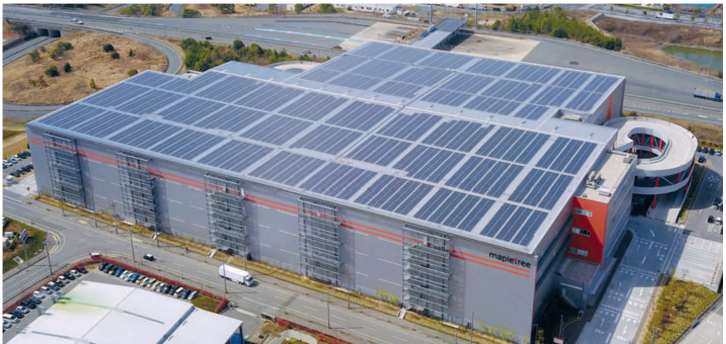
Rooftop solar panels at Mapletree Kobe Logistics Centre, Japan
