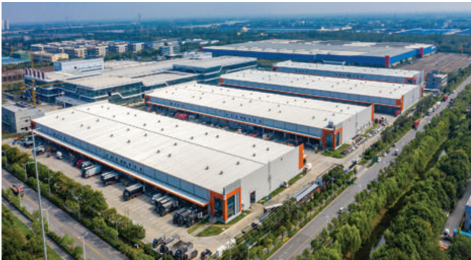
Mapletree Yangzhou Industrial Park
