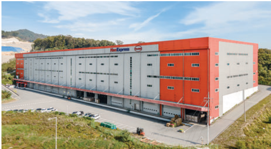
Mapletree Logistics Centre - Iljuk 2
