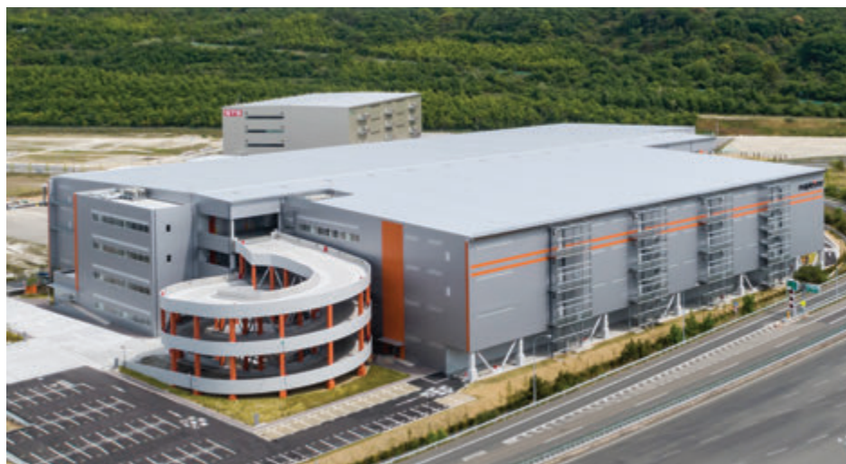
Mapletree Kobe Logistics Centre
