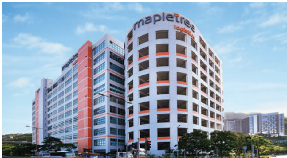
Mapletree Logistics Hub Tsing Yi
