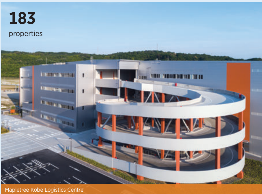
Mapletree Kobe Logistics Centre
